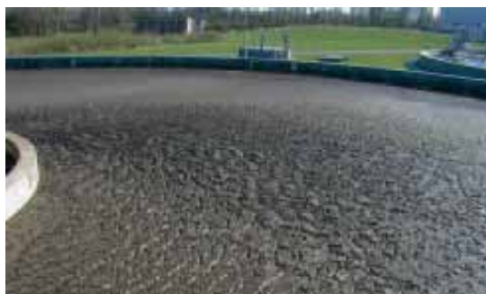
Figure 1 View of the final sedimentation basin with floating sludge
